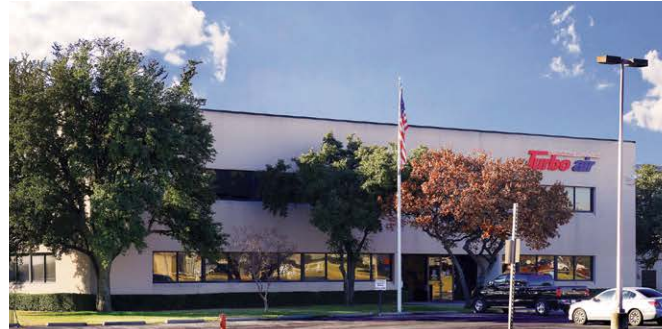
TEXAS, USA PLANT
